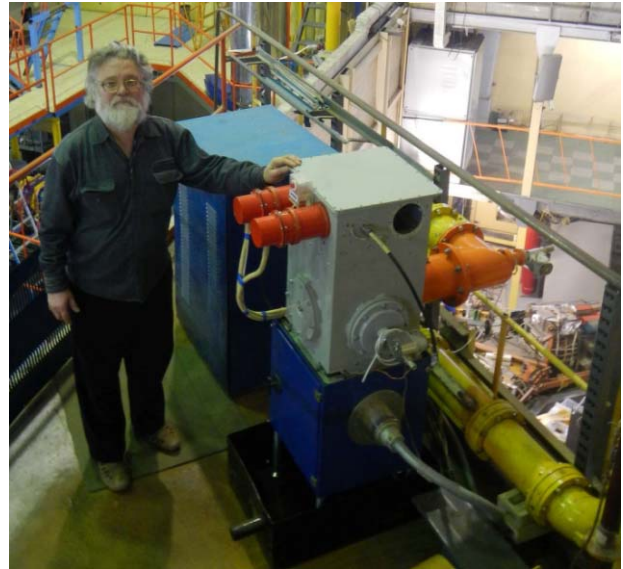
Fig. 7.5.2. Output stage of the BEP RF generator.
