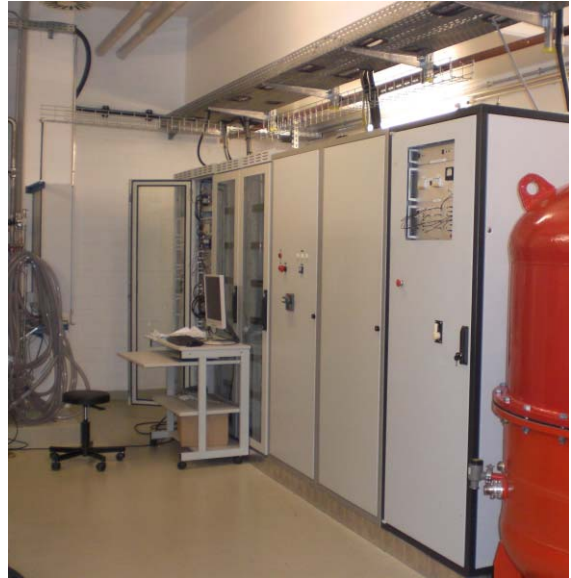
Fig. 7.2.1. HV PS for the diagnostics injector at RUDI-x.
