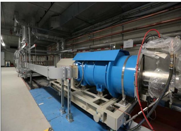
Fig. 5.7.4. First assembled SHF station of the XFEL injector (September 2013).
