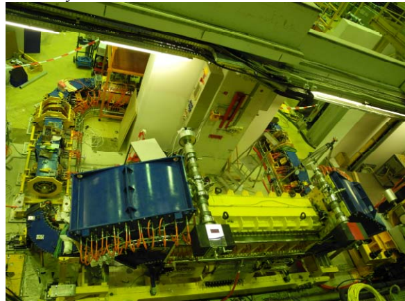
Fig. 5.9.3. Assembling the cooling section on the accelerator ring.
