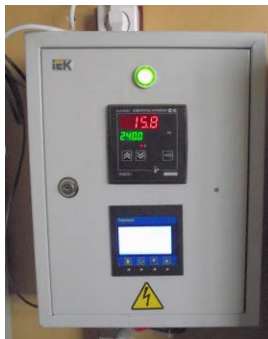
Fig.7.17.10. New controller for ovens.
