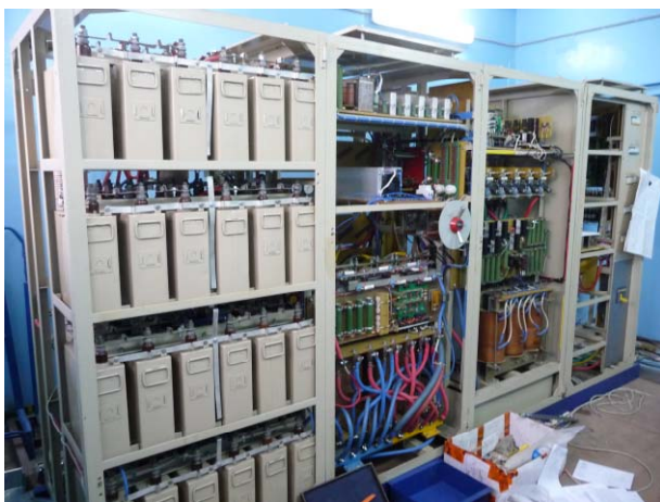
Fig. 8.1.2. ILU-10 power supply system for joint BINP-NSU laboratory.
