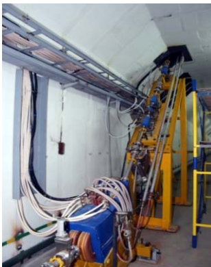
Fig. 5.2.12. Vertical section of the injection channel to VEPP-3.
