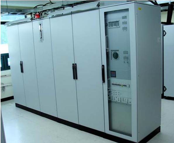
Fig. 7.11.1. Anode power supply (9.2 kV, 45 A).
