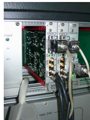
Fig.7.17.9. Control and measurement modules of GID-25PS.
