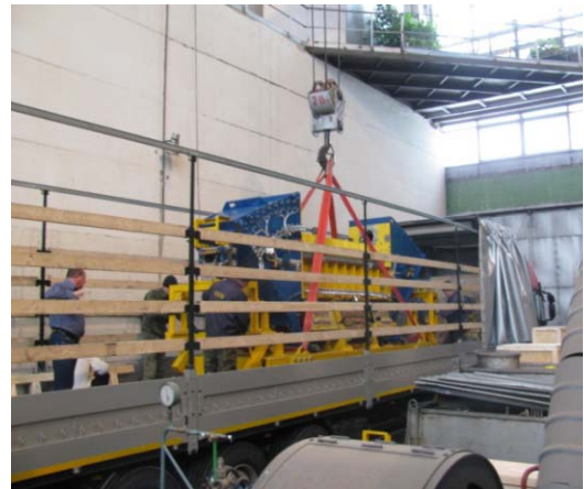
Fig. 5.9.2. End of 2012: loading of cooling section into a truck for transport to Germany.
