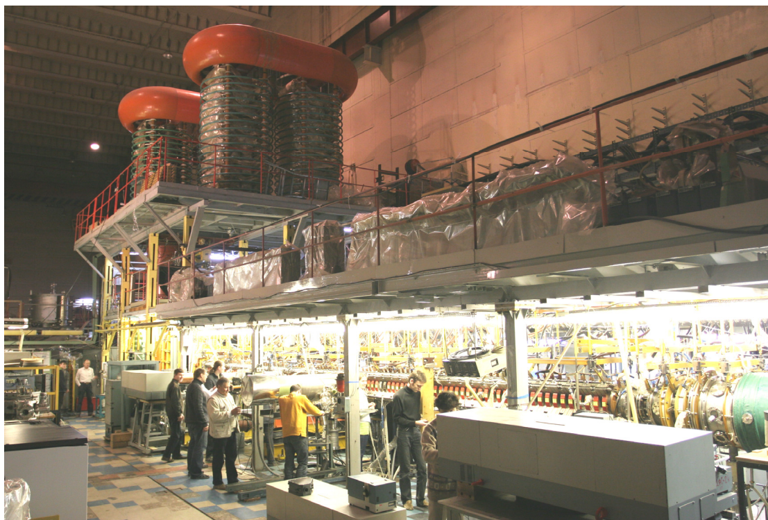
Fig. 4.2.1. Photo of the GOL-3 facility.
