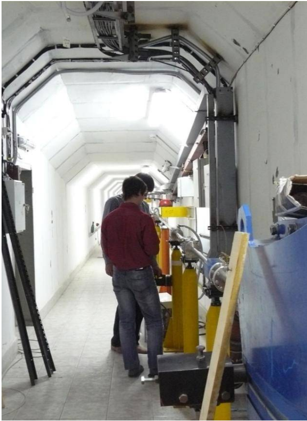
Fig. 5.1.13. Tunnel of K-500 channel.
