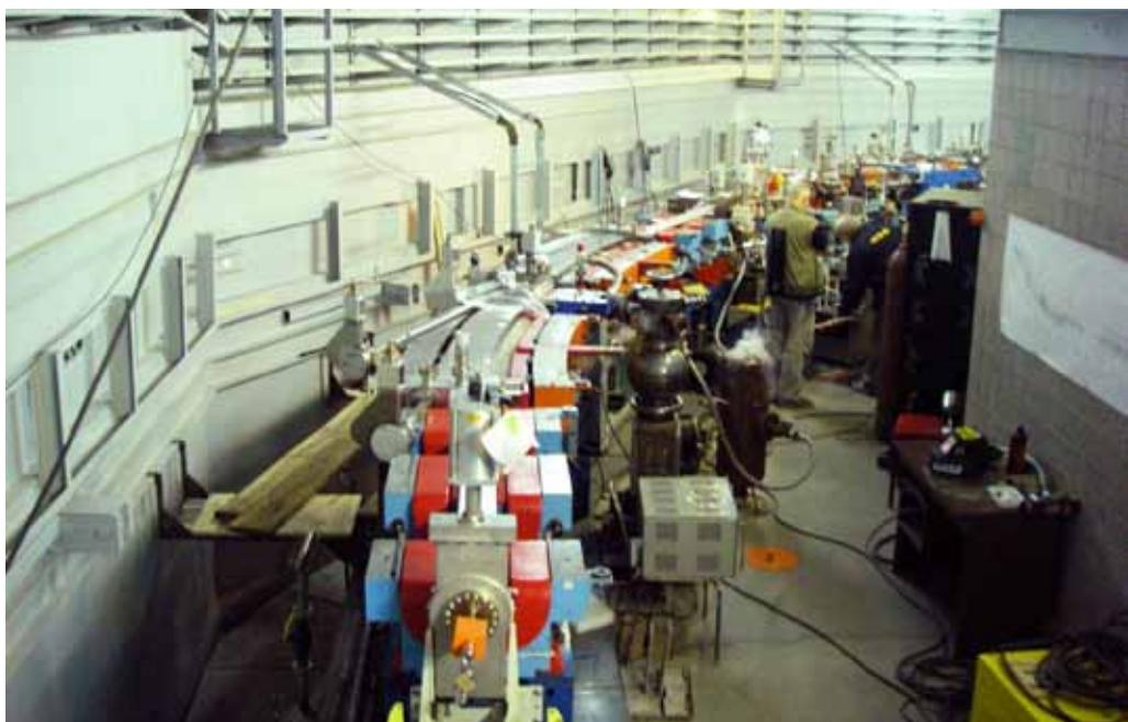
Fig.(6.4)3. Mounting the vacuum system of the large storage ring of SR source “Zelenograd”.
