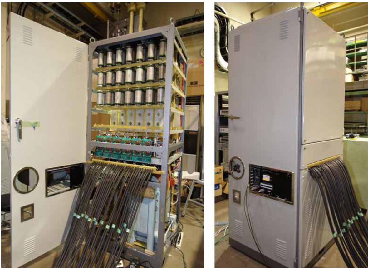
Fig.(5.13)1. Power supply of the conversion magnet.
