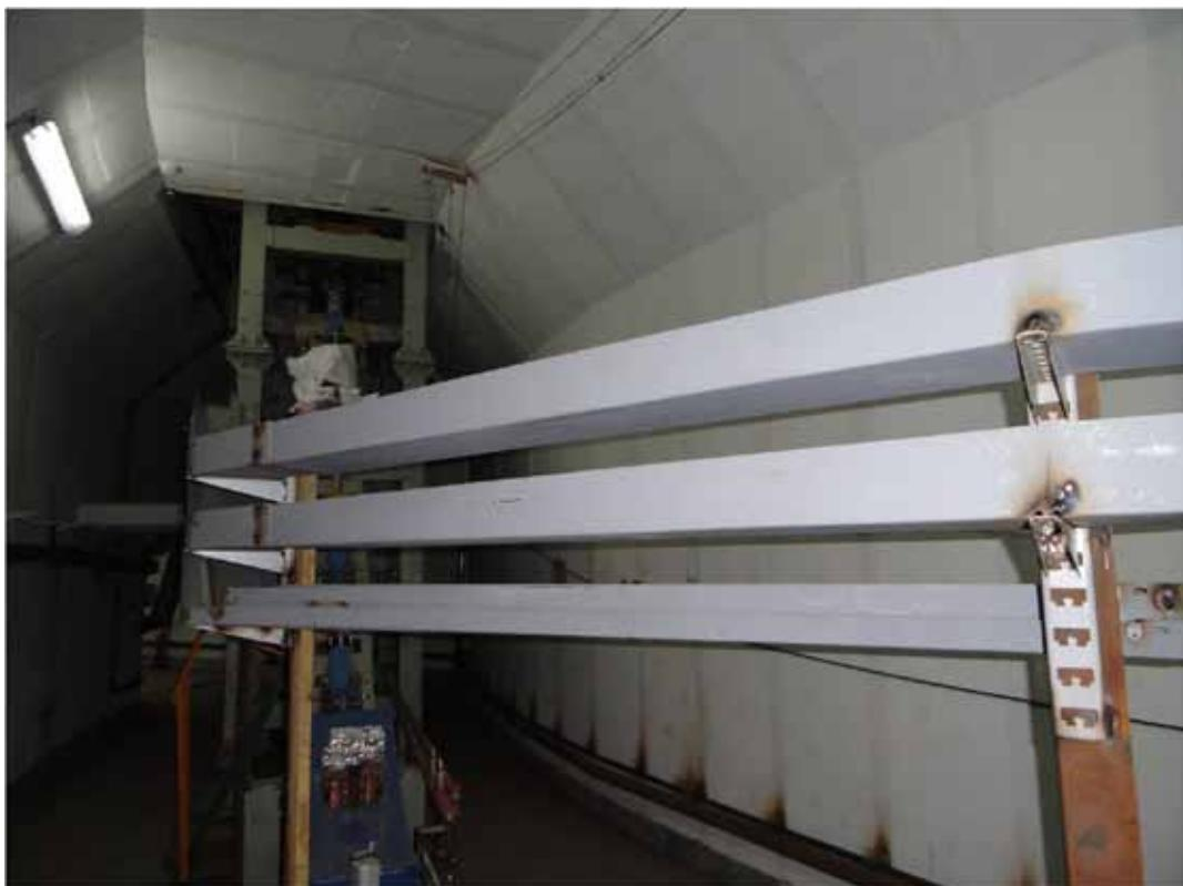
Fig. (5.3)8. Cable trays and ground loop at IC channel.
