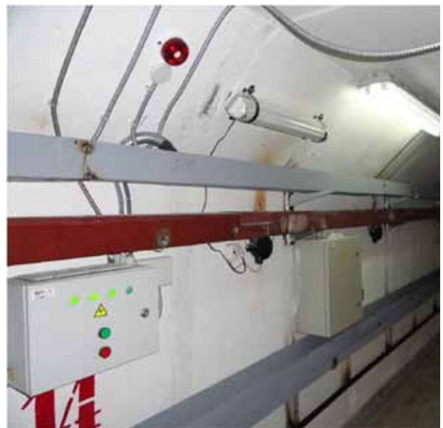
Fig. (5.3)7. The elements of fire alarm system at the channel of IC.
