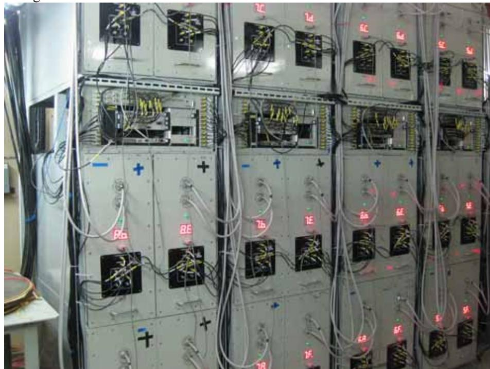
Fig. (5.4).1. High voltage modulators of LIA – 2 accelerator.
