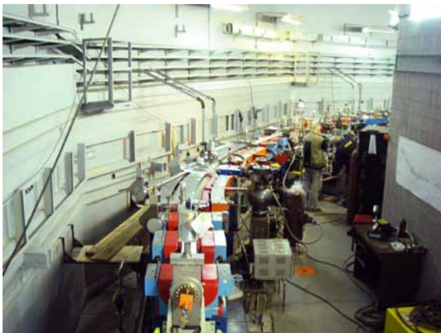
Fig. 39: Mounting the vacuum system of the LSR of the SR source “Zelenograd”.
