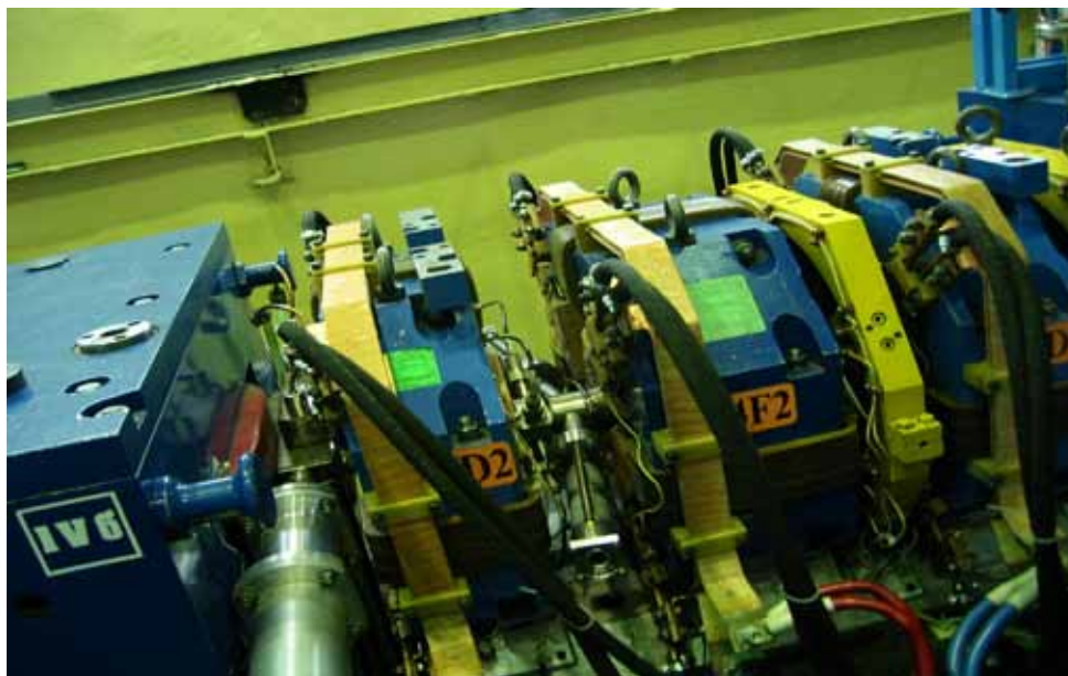
Fig. 4: Installed probes for particles registration.
