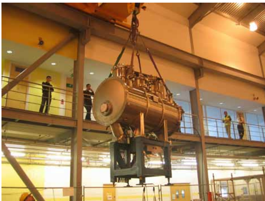
Fig. 32: Mounting the 49-pole wiggler with a field of 4.3 T on the DLS storage ring.
