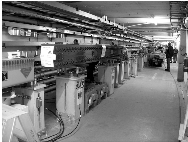
Figure 41: Installation of the wigglers in the straight sections of PETRA III.
