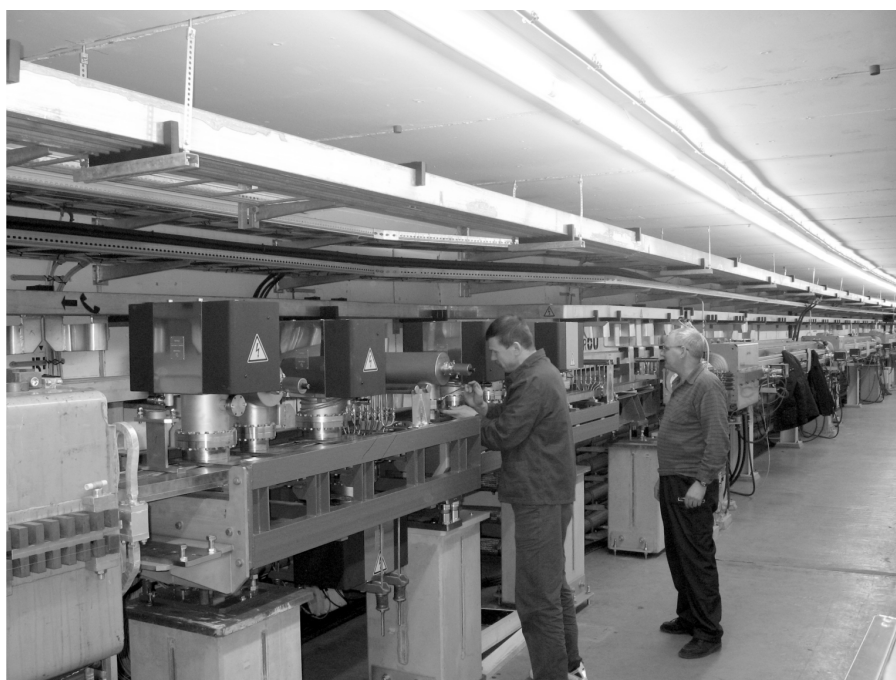
Figure 4: A 130 kW absorber. Assembly at PETRA III ring.
