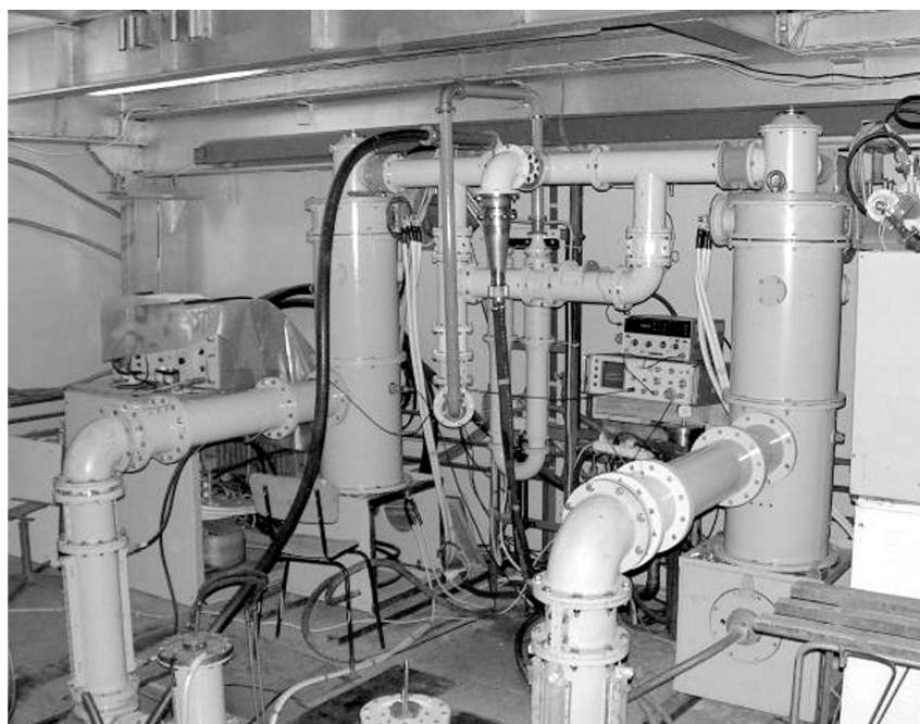
Figure 4: RF autogenerator on GI-50A triodes.
