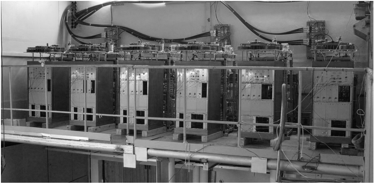
Figure 6: Overview of high-voltage part of new power supply system of GDT device (six of eight modules are shown).
